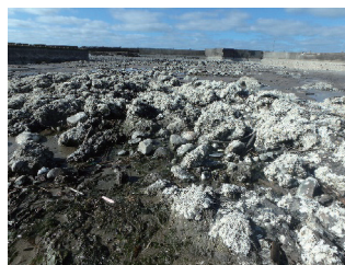
Fig.3 Ground upheaval in the harbor due to the Noto Peninsula earthquake
