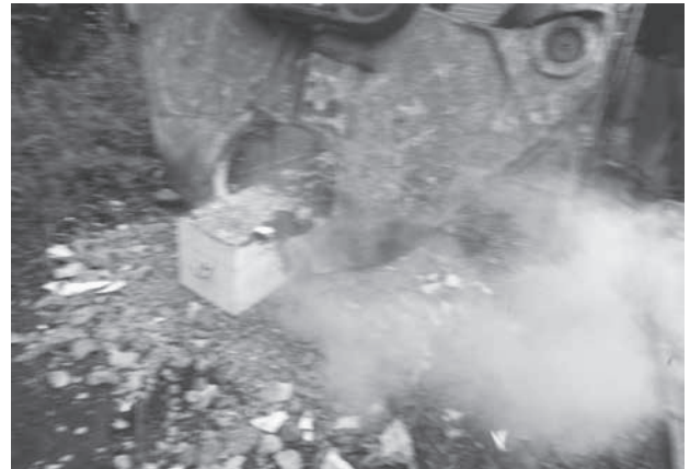
Fig. 12 Scatter of concrete pieces during crushing
