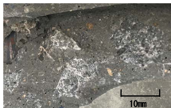
Fig.2 Tensile Crack of Aggregate.
