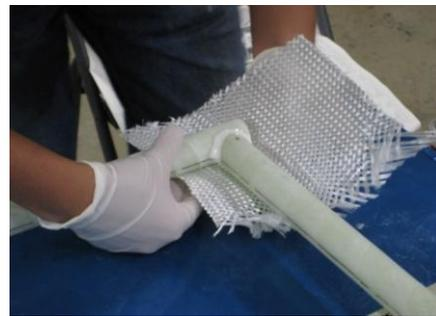
Fig.6 GFRP overlay process
