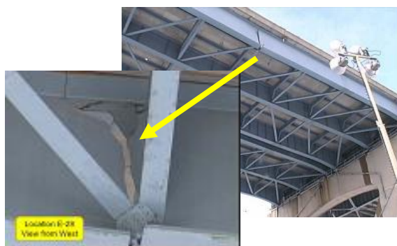
図-1 鋼橋の脆性破壊例 (The Hoan Bridge) 3)
