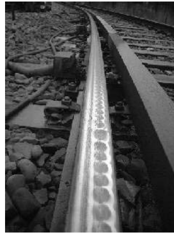
Fig. 1 Example of rail corrugation
