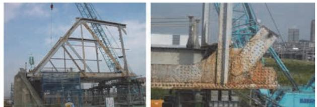
**Fig. 5 Dismantling of the 200ft plat truss girders**
