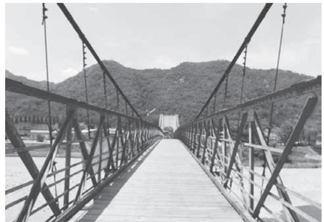
**Fig.14 Truss girders supported by main cables through hunger cables**
