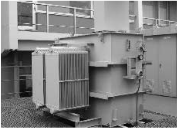
Fig. 5 Current-limiting reactor.
