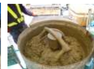
補修材練混ぜ
